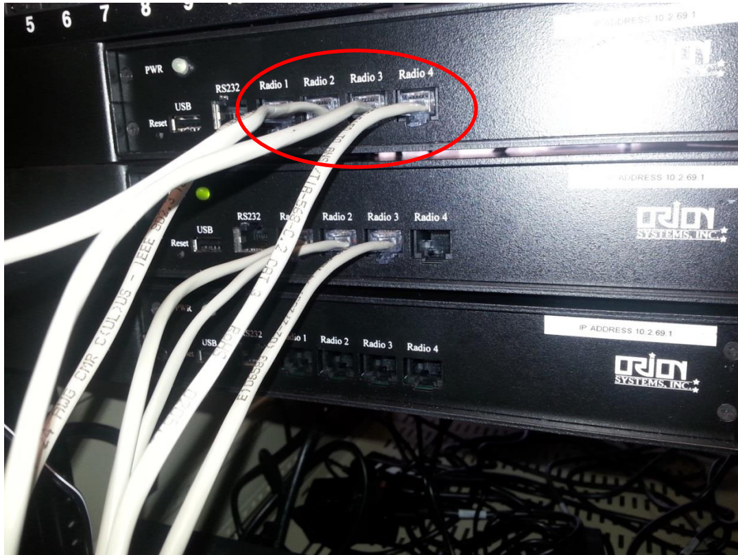
Exhibit 32.6-9 Connections to transmitters from failed DAC
